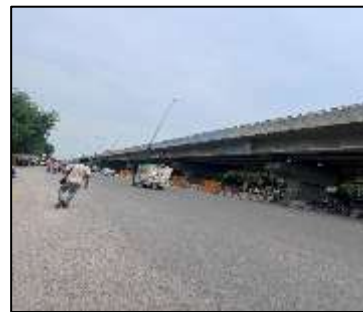
View of NH -48 (Secondary access road)
